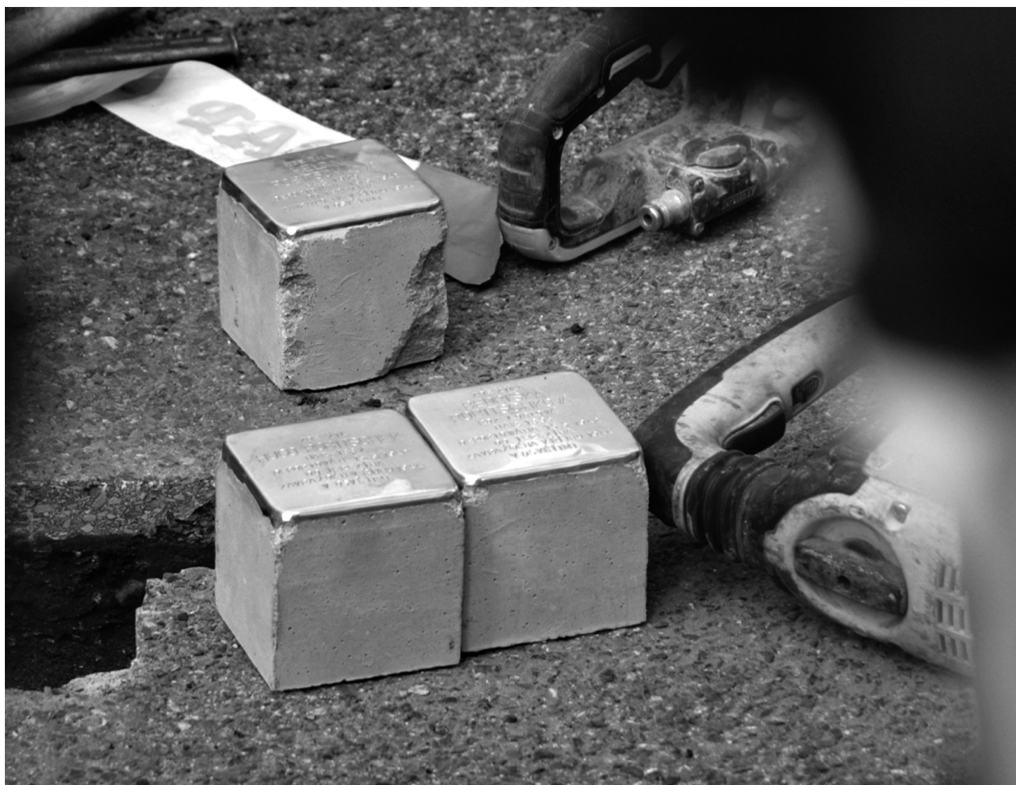
[Stolpersteine during their installation September 6, 2019]
