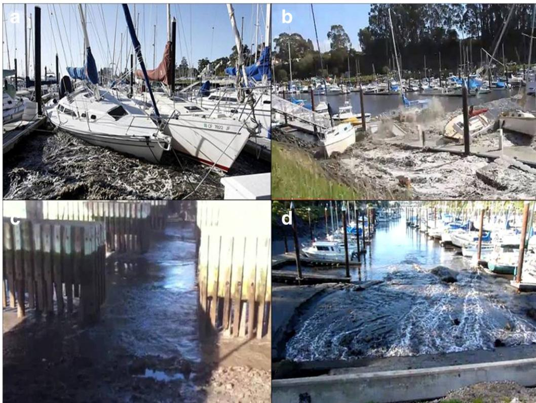
**Fig. 6.** Tsunami currents, erosion, and damage in Santa Cruz Harbor. (a) Strong currents cause damage to boats within harbor; (b) heavily damaged or destroyed docks as tsunami bores enter the northern part of the harbor; (c) base of bridge foundation exposed and scoured as receding waters rush through the central part of the harbor; (d) scour where drainage from Arana Gulch Creek enters the harbor at the north end.
