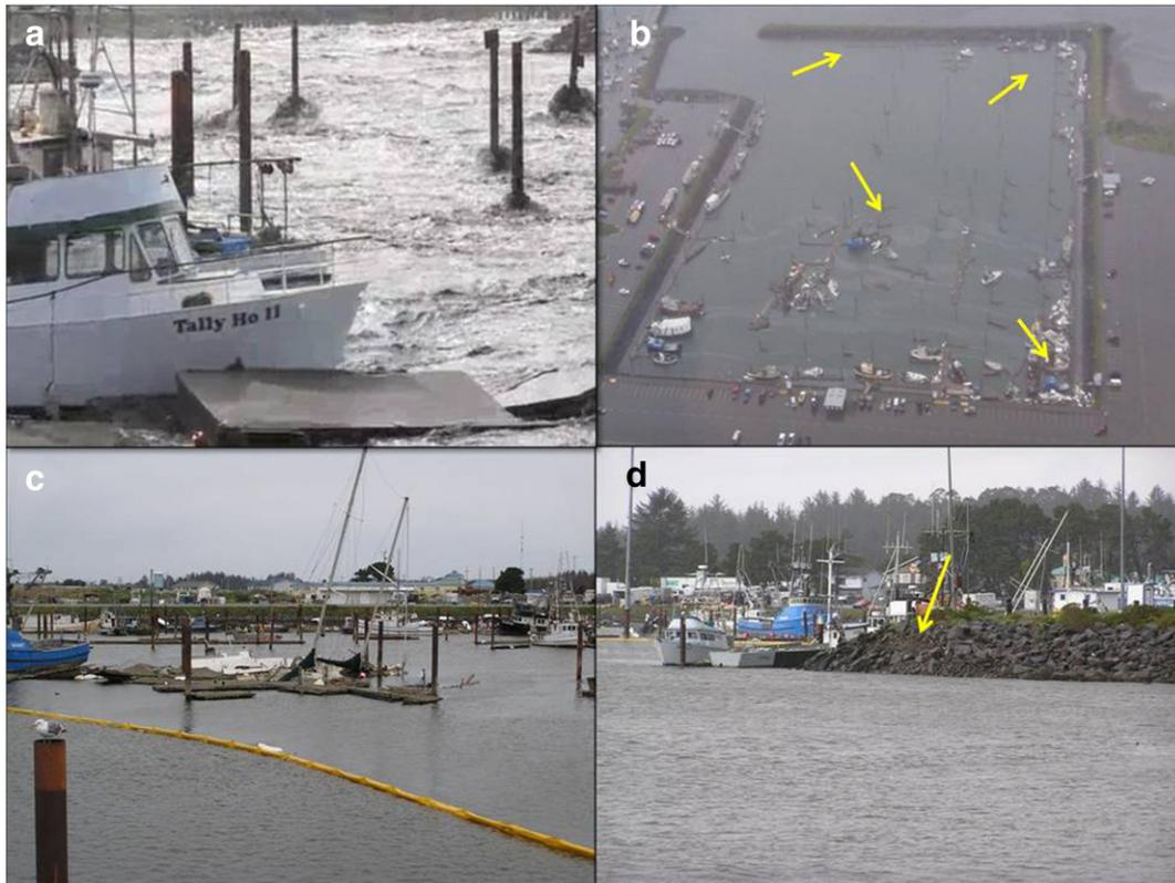
**Fig. 2.** Tsunami currents and damage in Crescent City Harbor. (a) Strong currents at the mouth of the Small-Boat Basin and across the center of basin; (b) heavily damaged or destroyed docks. Yellow arrows show areas of sediment accumulation; (c) sunk boat sits on shallow floor of Small-Boat Basin where sediment has accumulated; (d) failure of slopes caused by tsunami scour and undercutting.
