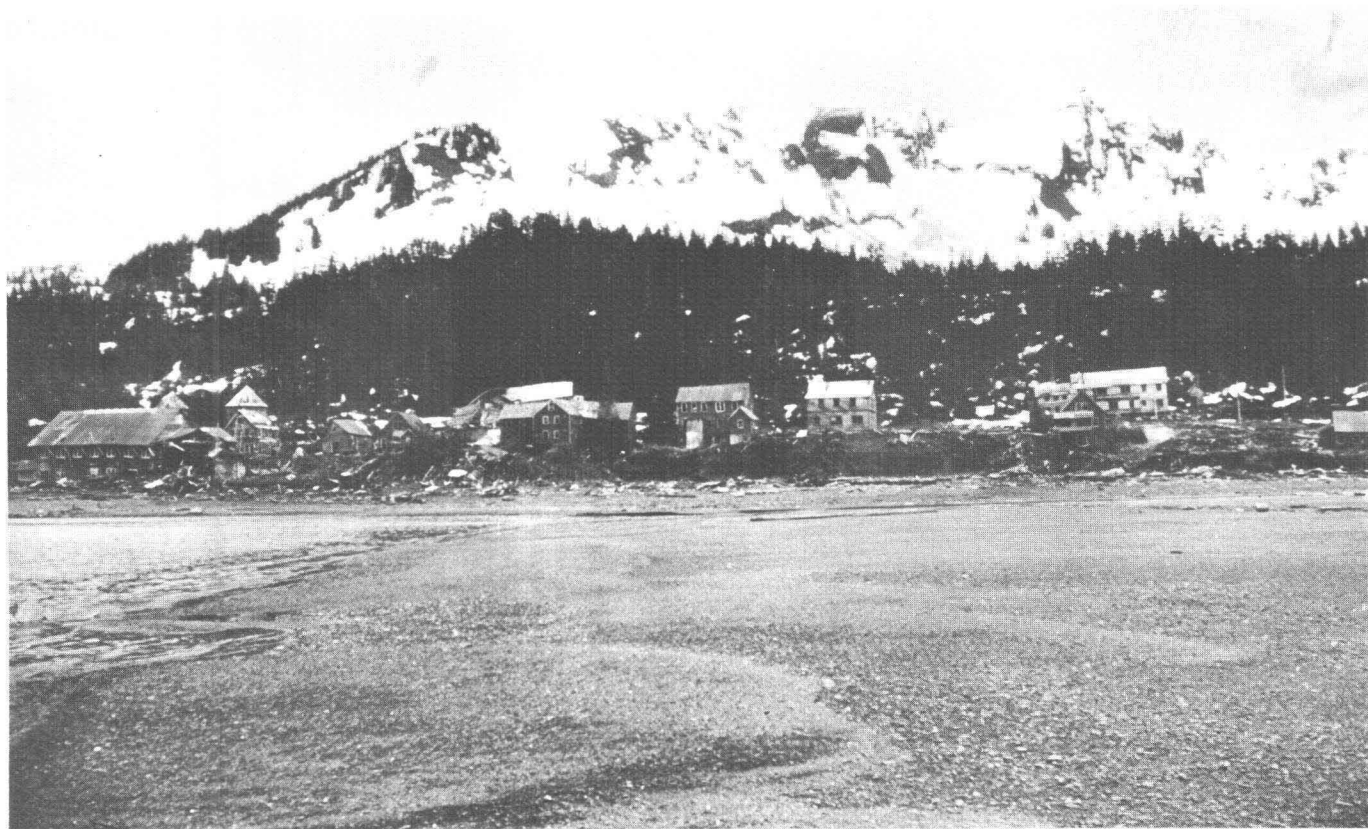
13.—Remains of buildings partially damaged by waves along part of Latouche waterfront. Docks, piers, and some buildings in this area were swept away. Approximately 11 feet of tectonic uplift has raised this former port above the reach of most tides.
