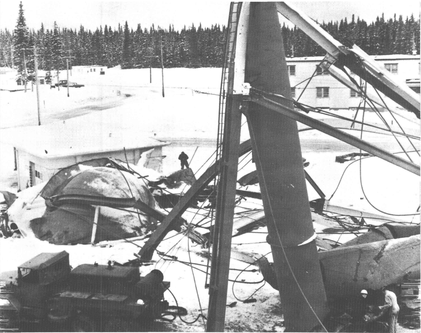
25.—View westward showing southwest half of collapsed water tower at Wildwood Station. Officers' club in background. Photograph by U.S. Air Force.
