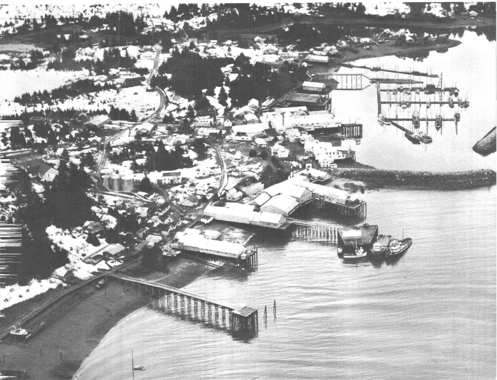
30.—Seldovia as it appeared in March 1965, with restored inner harbor facilities and breakwaters, piers, and docks raised to compensate for the 3½-foot tectonic subsidence. Photograph by U.S. Army.
