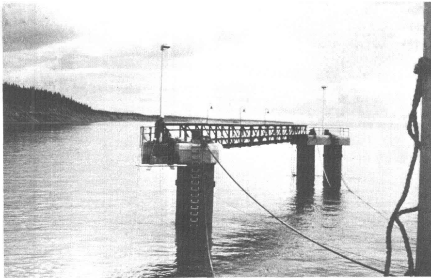
27.—Collapsed catwalk at Nikiski refining facility.
