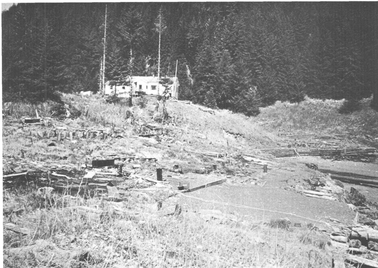
6.—Main part of the Chenega village site. Piling in ground marks the former locations of homes that were swept away by waves. Schoolhouse on high ground was undamaged.
