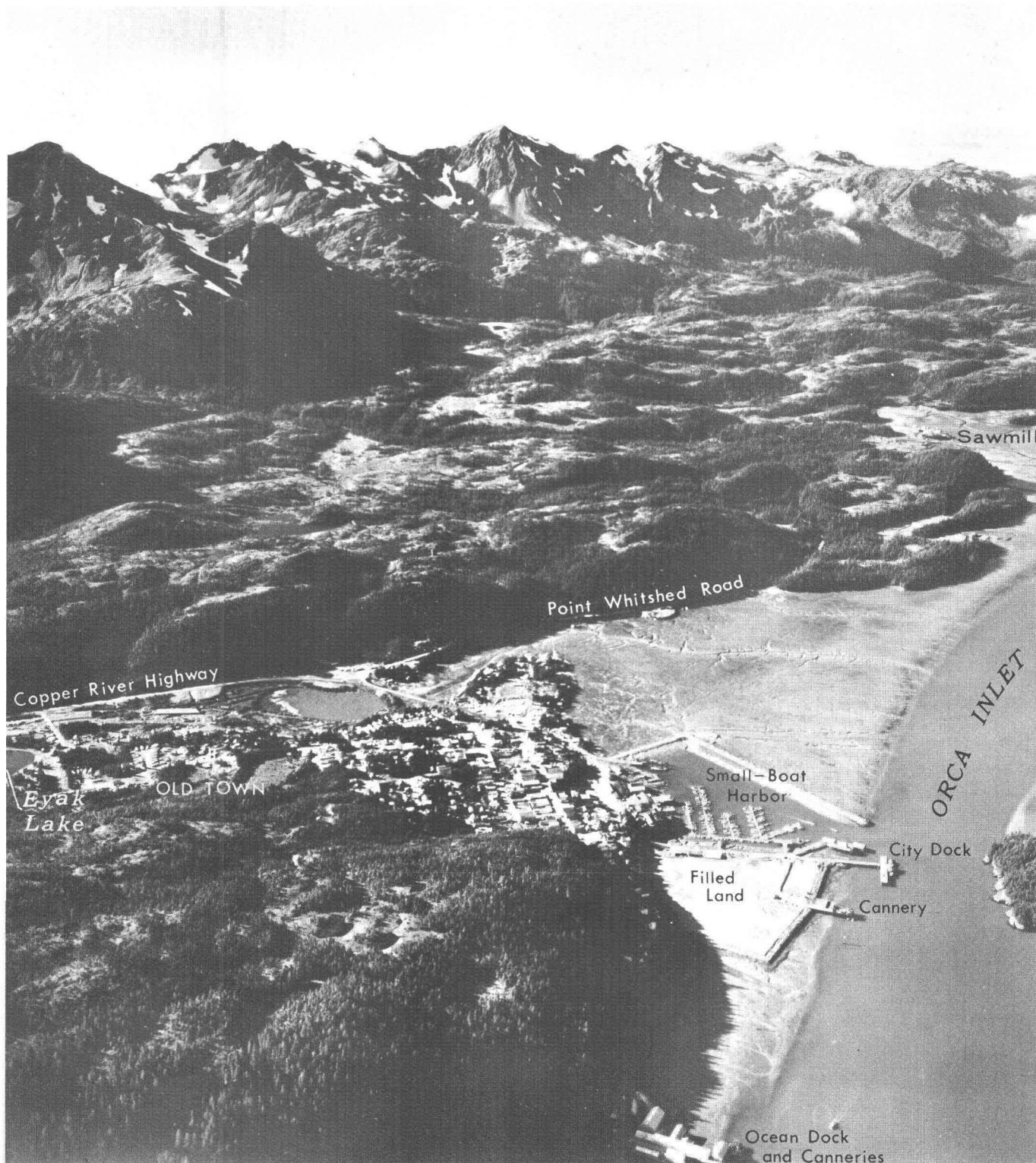
S.—Cordova, as it appeared in September 1966, with port facilities rebuilt to compensate for the 6-foot tectonic uplift of the shore-line. Looking south, with end of Eyak Lake and Copper River Highway in left center, and Cordova sawmill, destroyed by seismic sea waves, toward upper right. The white angular patch, lower right, is new land made from material dredged from the deepened and enlarged small-boat basin. Photograph by U.S. Army.
