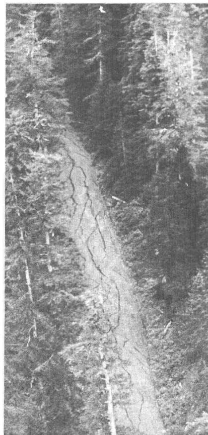
24.—Intensely fissured road at the crest of an elevated beach ridge west of Yakataga.
