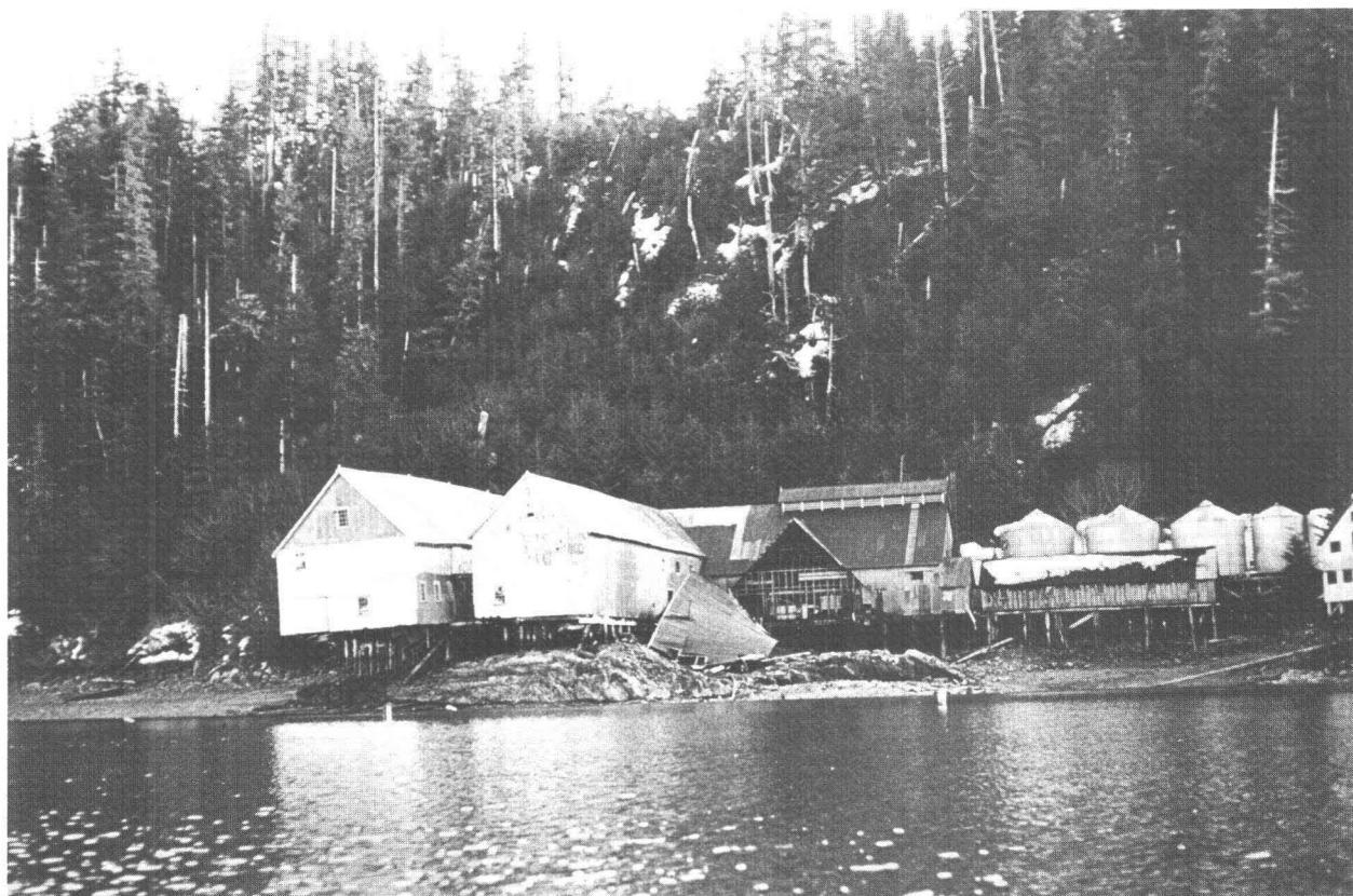
18.—Buildings at the Port Oceanic cannery damaged by a wave that struck within 2 to 3 minutes of the initial shock and had a crest height about even with the cannery floor level. Photograph taken April 4, 1964.
