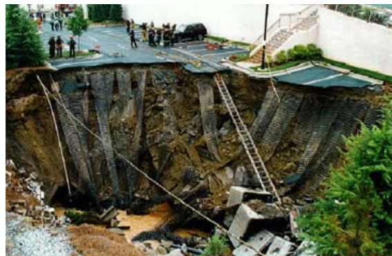
Collapses, such as the sudden formation of sinkholes, may destroy buildings, roads, and utilities. (Photo: Bettmann)
