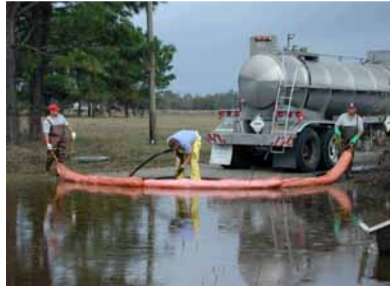
Propane tanks, gasoline, oil and other hazardous materials and debris in Princeville, North Carolina were cleaned up by Environmental Protection Agency crews following Hurricane Floyd in September 1999. The town remained off limits to residents for some time due to health-related concerns. (Photo by Dave Saville/FEMA News Photo)
