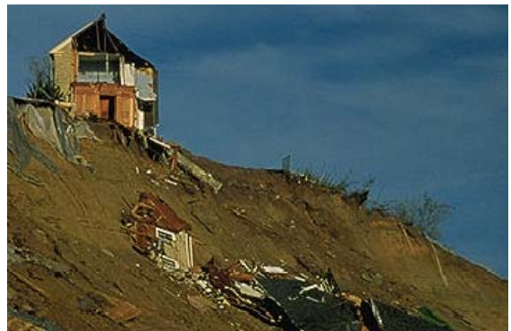
Landslides can damage or destroy roads, railroads, pipelines, electrical and telephone lines, mines, oil wells, buildings, canals, sewers, bridges, dams, seaports, airports, forests, parks, and farms. (Photo by Lynn Forman)
