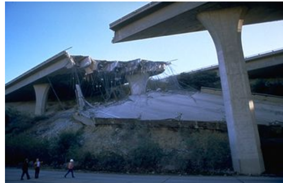
Many roads, including bridges and elevated highways, were damaged by the 6.7 magnitude earthquake that impacted the Northridge, California area January 17, 1994. Approximately 114,000 structures were damaged and 72 deaths were attributed to the event. Damage costs were estimated at $25 billion. (FEMA News Photo)
