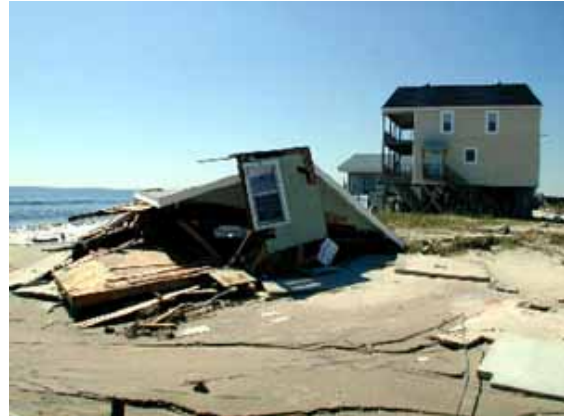
Hurricane Floyd brought a devastating 15 feet of storm surge that damaged or destroyed hundreds of houses along the ocean front of Long Beach on Oak Island, North Carolina in September 1999. A prime example of successful hazard mitigation, the elevated home (right) survived while the older, ground-level block foundation of the home on the left was crushed. (Photo by Dave Gatley/FEMA News Photo)
