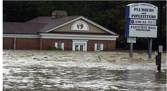
Flood waters rush by the Faith Harvest Worship Center on Del. 4 near Newport during flooding that occurred September 18, 2003, largely as a result of remnants of Tropical Storm Henri. (Photo courtesy of The News Journal/Ginger Wall)
