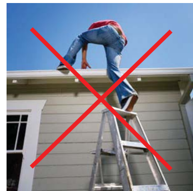
This picture demonstrates exactly how NOT to use a stepladder
