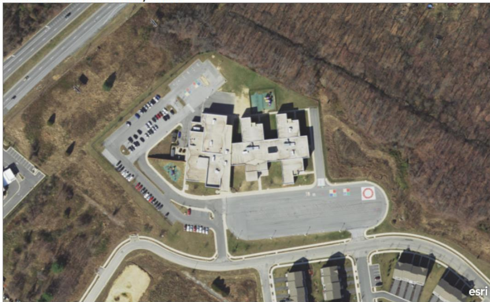
An aerial view of Oberle Elementary School in Bear, DE. Used for a DTI unit.
