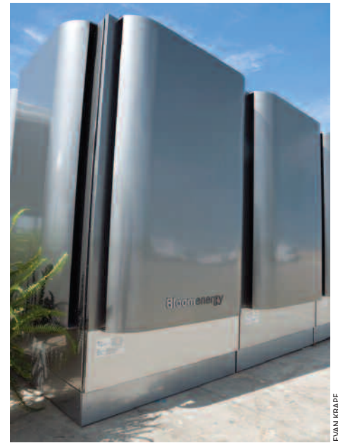
Bloom Energy servers convert natural gas into electricity. Groundbreaking for Bloom's first East Coast manufacturing center took place in April for this first tenant of the STAR Campus.
