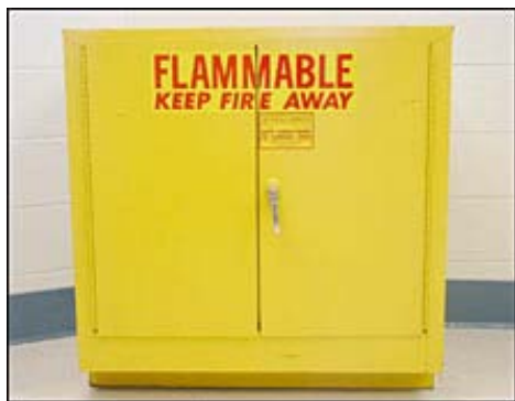
Store flammable combustible liquids in rated flammable cabinets.
