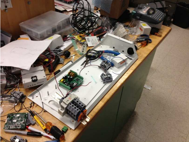
(a) Initial work on three-phase EVSE. Initial work on three-phase EVSE. It required modifications to all line power components, and the DC power supply, for three-phase, 400/480V capability.
