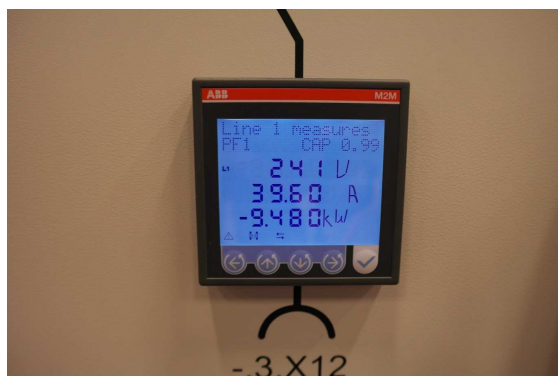
(f) Discharge at 40A, 9.5kW
