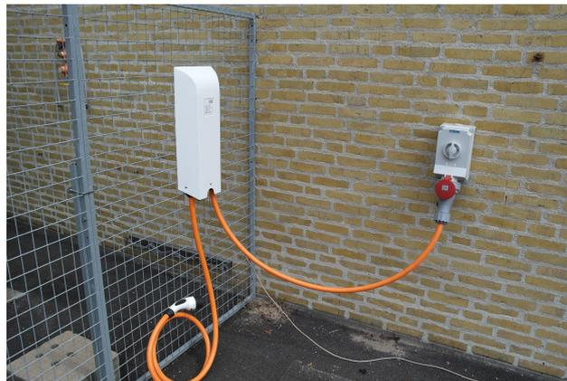
(d) Temporary EVSE installation for testing. It draws 63A from a CEE outlet.
