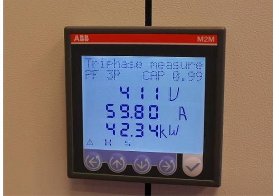
(b) Panel meter measures charge rate to 42.3kW with 0.99 power factor.
