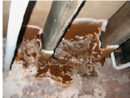
Dry Rot on the underside of the basement floor
