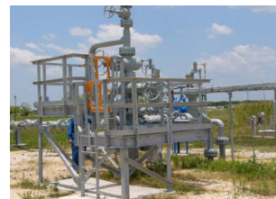
Outlet valve of a hydrogen cavern
