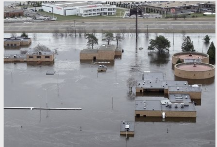
Cranston WWTP (Rhode Island) March 2010 Damage: $10 million Photo: Providence Examiner
